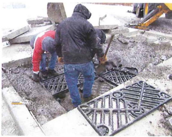
Manual removal of two decks, unscrewed and set aside for future re-installation.
