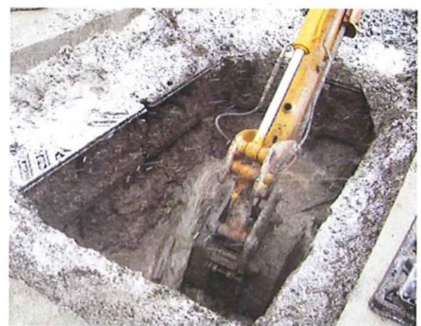
Excavation below bottom of soil cells to daylight water pipe.
