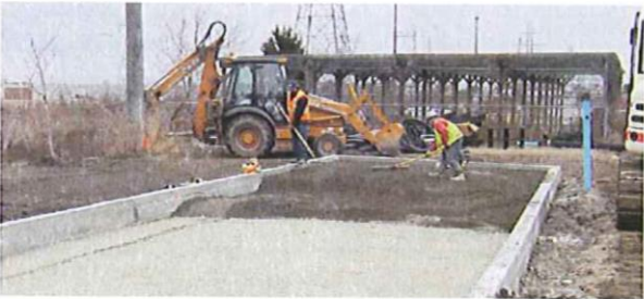
Backfill installation on top of deck.
