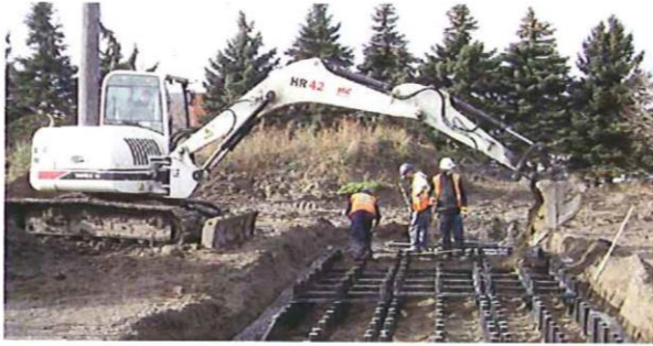
Soil cell trench filled with soil
