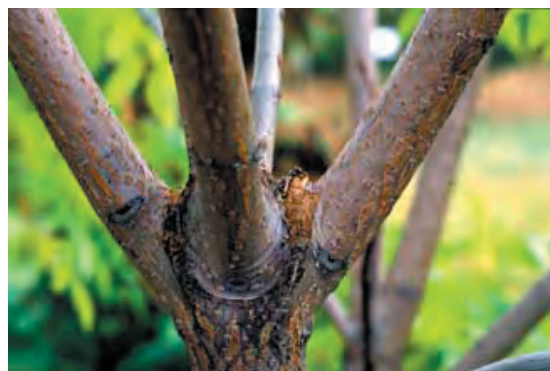
Figure 4.4. Avoid purchasing nursery stock with codominant leaders (more than one leader), or select stock that can be successfully pruned back to a single leader. Even though these branch attachments are not weak, this codominance began 3 feet above ground, far too low for a tree that will mature to 40 to 50 feet in height.
