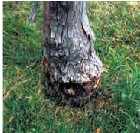
Figure 4.1. Lawn mower and string trimmer damage caused by mechanical injury and subsequent decay at the base of the tree.
