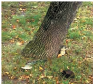
Figure 3.81. A leaning tree that also had advanced decay in the root collar.
