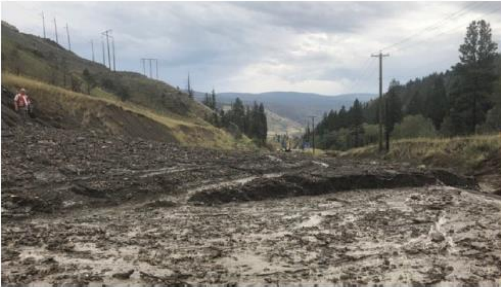
Figure 2-4. Debris flow blocking Highway 97 south of Clinton, BC on July 31, 2018 (MOTI, 2018). This area was burned in 2017 by the Elephant Hill Wildfire.
