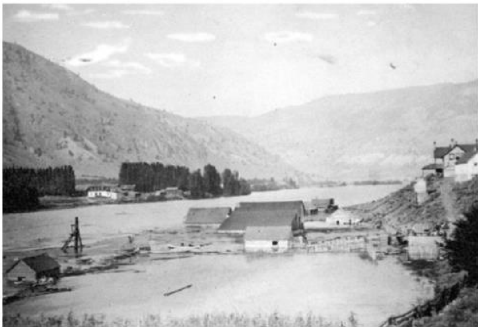
Figure 5-1. Upstream flooding caused by a landslide dam near Spences Bridge in August 1905 (Cooks Ferry Band, 2015).
